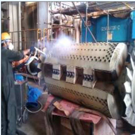
35MVA, Alternator Rotor Cryogenic Cleaning
