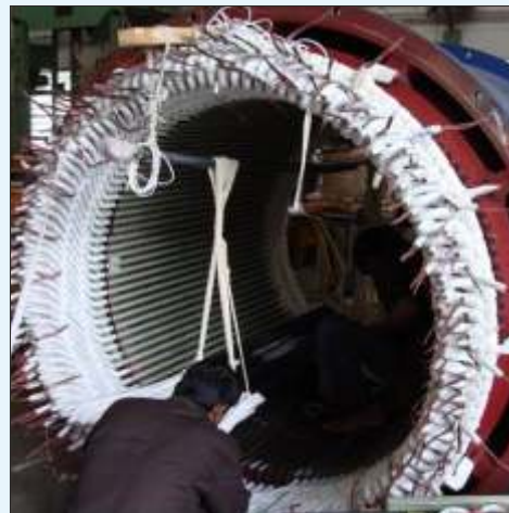
8MVA,11KV, Alternator Stator Rewinding
