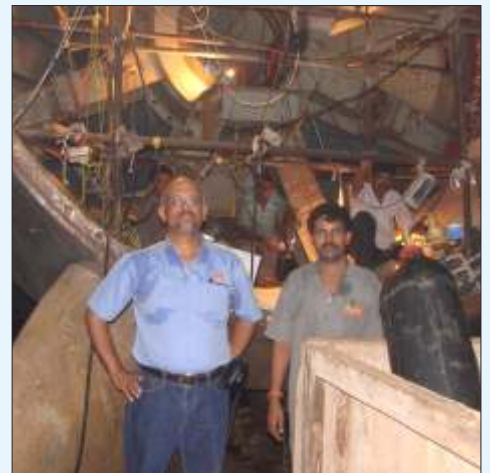
6MVA, Stator Rewinding Under Progress
