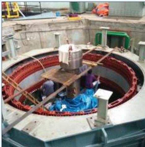
11.25MVA, 11KV Alternator Overhauling
