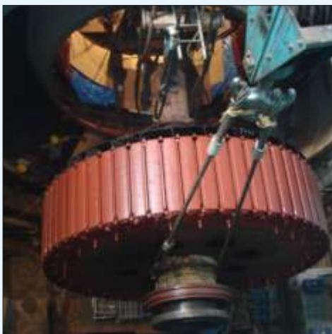
6MVA, Rotor Threading In
