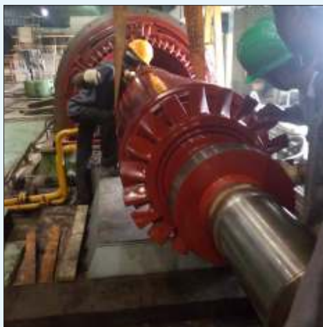
8MVA, Alternator Rotor Threading In
