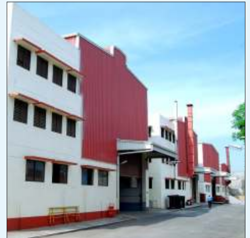
Plant At Tumakuru
