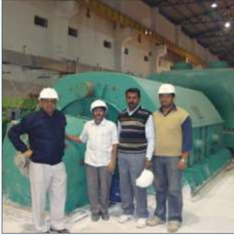
61MVA, Alternator Post Overhauling
