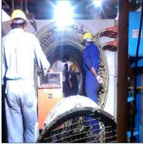
35 MVA, Stator, Cryogenic Cleaning
