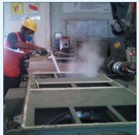
1MW, Stator Cryogenic Cleaning
